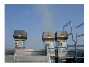
The chimney fan itself is mounted at the top of the flue, on the roof of the tower block, to control the draught in the flue and maintain it at the most fuel-efficient and energy-efficient level possible. Electronic controls sense the fluctuating flow of gases in the flue as the number of boilers firing rises and falls, and control the speed of the fan, and thereby the upward flow of flue gases, appropriately to conditions in the flue.
